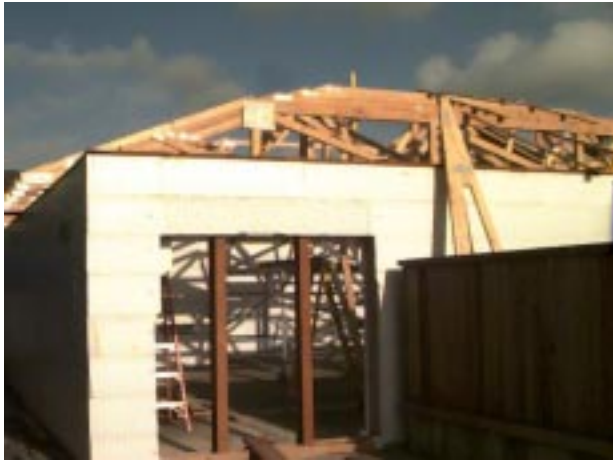
New Seawater Building
