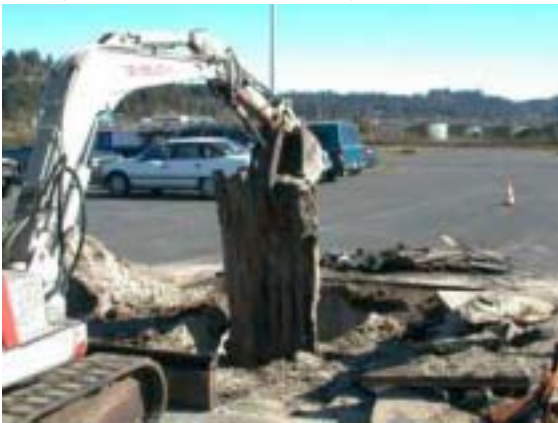
Backhoe plucks out log
